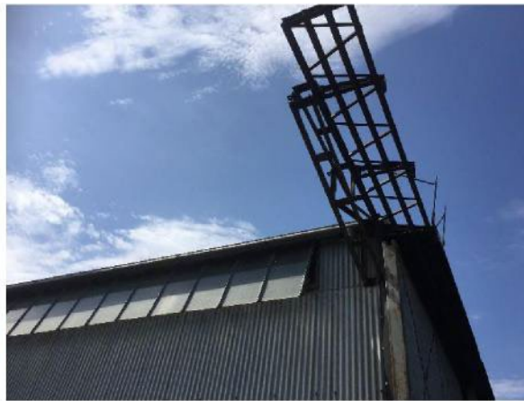
Figure 3.22 Clerestory side fixed sash lights glazed with wired glass. (Source: GML, 2018)
