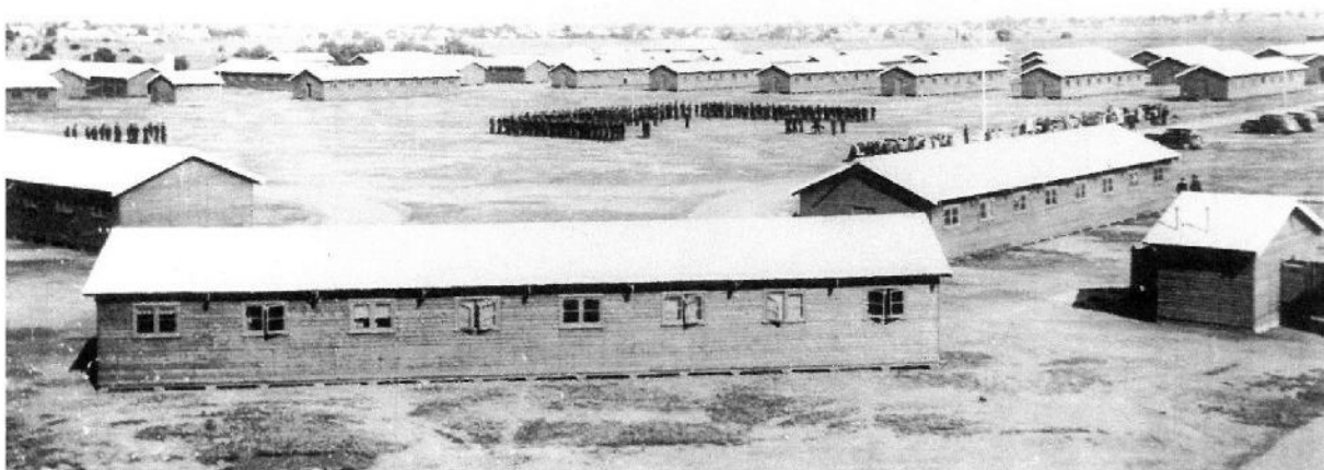
Figure 2.6 View from duty pilot's tower southeast over the base c1940. The headquarters building is in the foreground, the parade ground in the midground with the airmen's and trainees' quarters precinct in the background. (Source: Norma Meadley, Narromine History Room)
