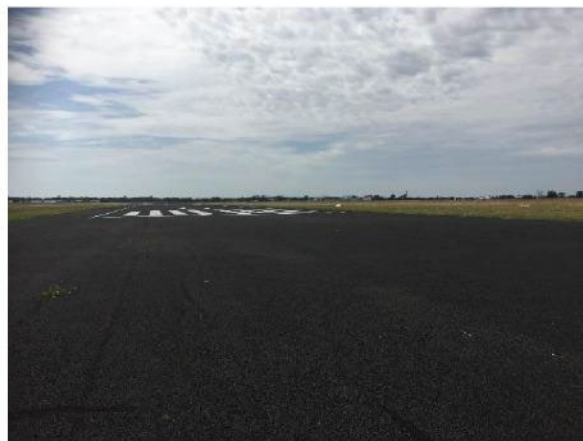
Figure 3.5 Paved runway in the airfield. (Source: GML, 2018)
