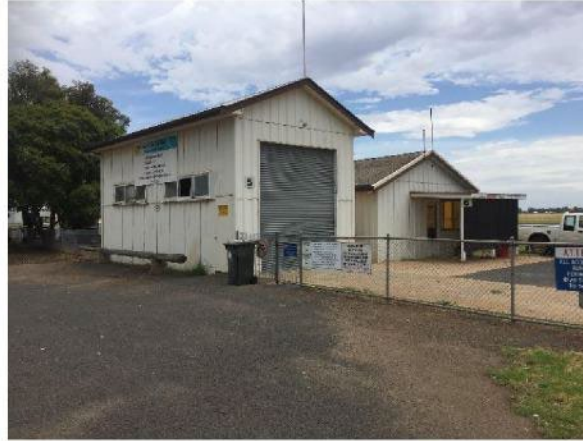
Figure 3.34 Building 5 (left) and Building 6 (right). (Source: GML, 2018)
