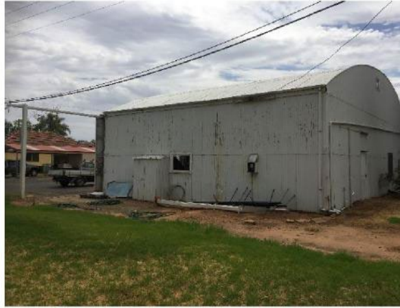
Figure 3.12 Side and rear of Hangar No. 1. (Source: GML 2018)
