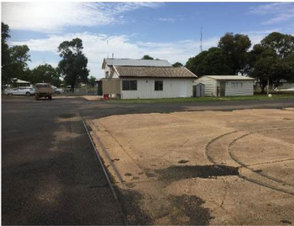
Figure 3.35 Buildings 5, 6 and 7 with the concrete slab of removed Bellman in foreground. (Source: GML, 2018)
