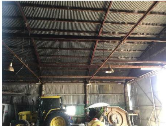
Figure 3.14 Steel roof framing of Hangar No. 1. (Source: GML, 2018)
