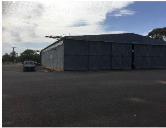
Figure 3.18 Western side of Bellman Hangar. (Source: GML 2018)
