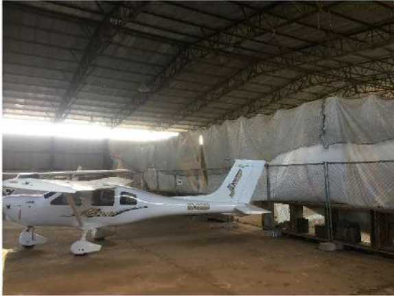
Figure 3.19 Interior of Bellman Hangar. (Source: GML, 2018)
